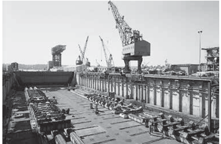
Dry Dock 3 at PSNS showing caisson (background) and wall.
