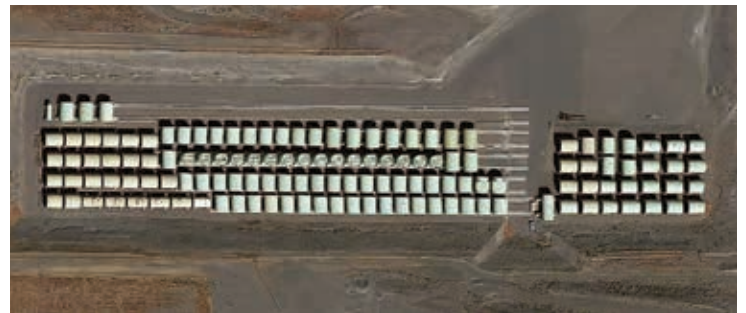
Area 200, Trench 94, Hanford Works.
